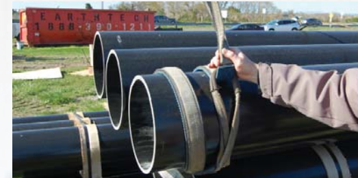
Lift-It® Sling Double Wrapped Around SUPERPILE
