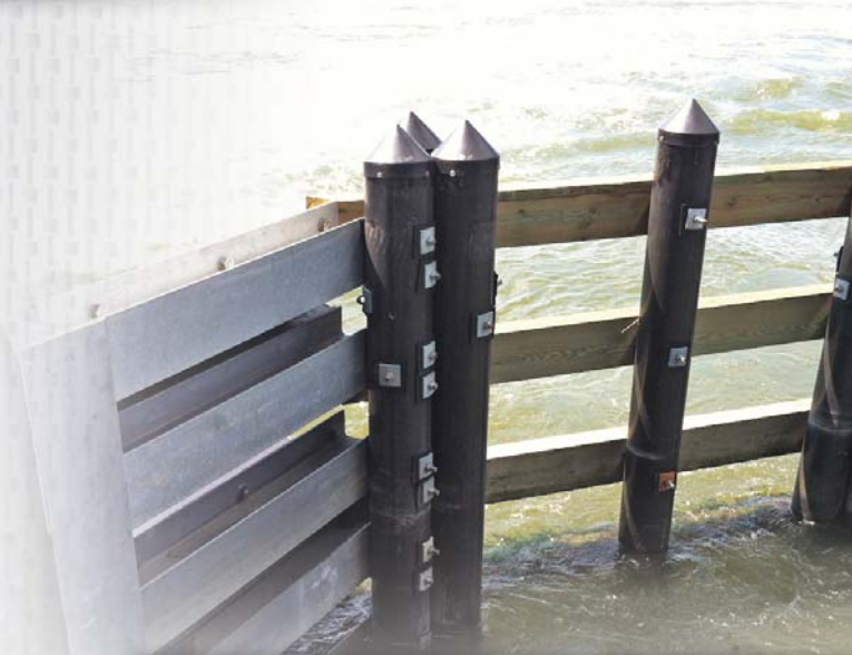
Margate Bridge Installation, Margate New Jersey
