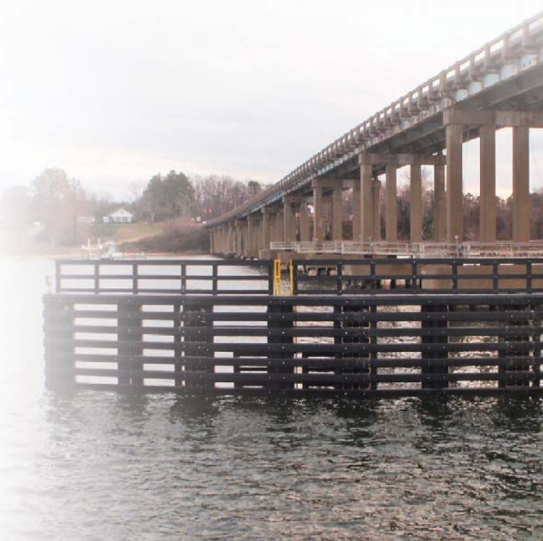
Fender Rehabilitation Route 3 Over Piankatank River, Virginia
