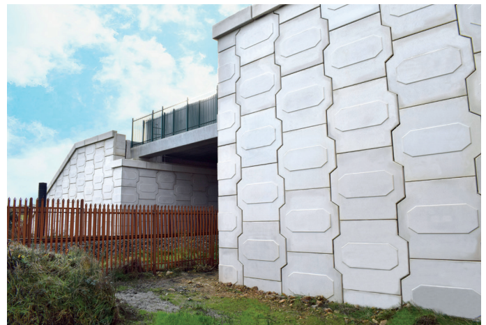
M11 Rail Bridge Scheme – Asset International Structures asset VSoL Cross Panel.
