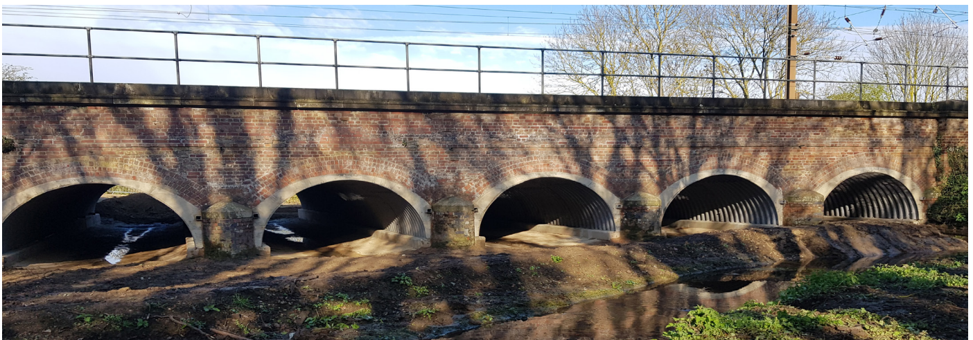
asset MultiPlate® MP200 Lolham - Rail viaduct near Peterborough
