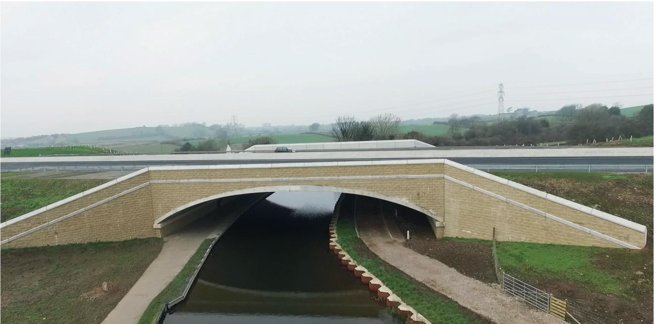
Heysham to M6 Link - Milestone Canal Bridge(654BI) (BEBO Arch T94S - Span 28.651m - Rise 3.213m)
