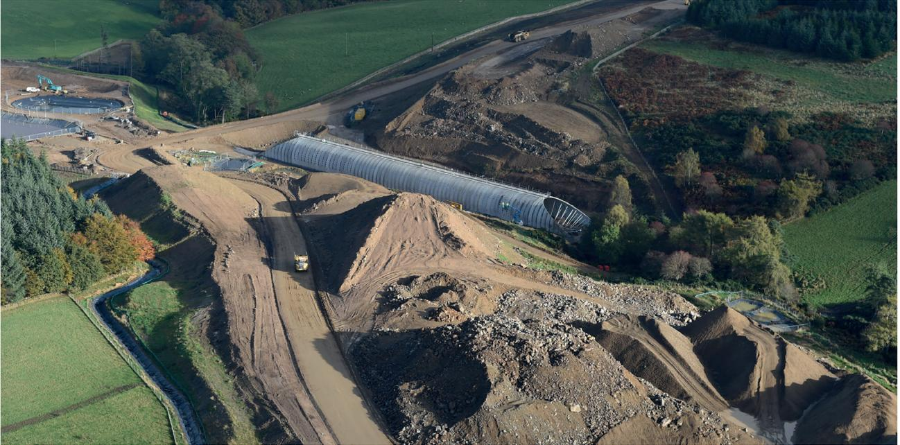
Aberdeen Western Peripheral Route PS02 and PS41A (BEBO Arch C42T/9 - Span 12.802m - Rise 8.026m)
