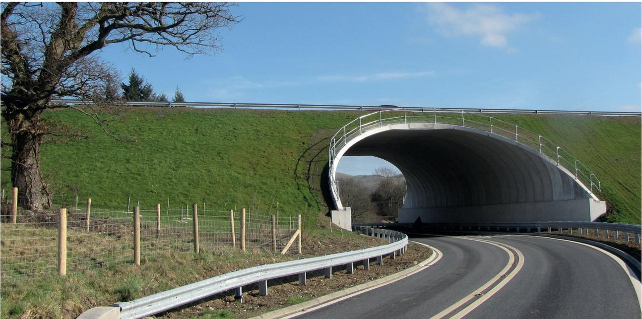
A470 Cwmbach to Newbridge -on-Wye- Red House Bridge (BEBO Arch E15.5Mt/5 - Span 15.5m - Rise 5.6m)
