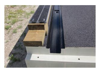
Drainage trench is moulded into the panel surface near the back edge of the panel. Grating covers the trench. The rainwater down pipes will be spaced at agreed centres and fixed to the underside of slab.
