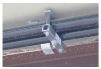
Hangars on the bottom of the deck carry utilities and conduit.
