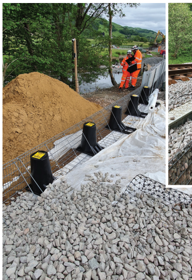
Black Bridge Machynlleth Supplied asset BaFix® 70 and Sleeve-It
