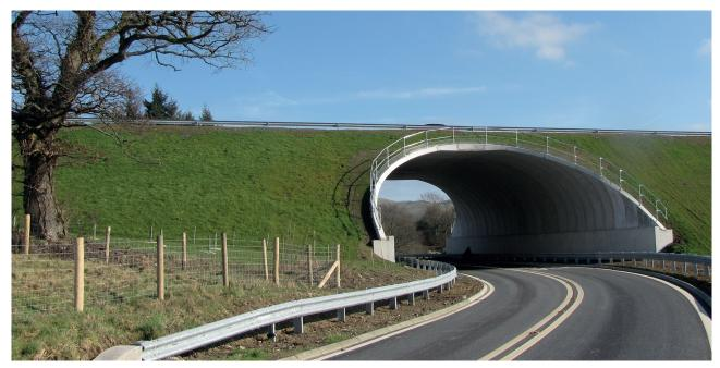
A470 Cwmbach to Newbridge -on-Wye- Red House Bridge (BEBO Arch E15.5Mt/5 - Span 15.5m - Rise 5.6m)
