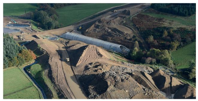
Aberdeen Western Peripheral Route PS02 and PS41A (BEBO Arch C42T/9 - Span 12.802m - Rise 8.026m)
