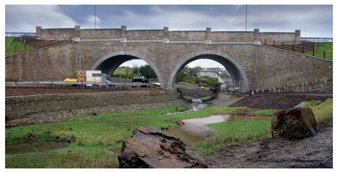
Camborne Pool - Redruth East - West Link - Red River Valley Arches (BEBO Twin Arches C42T/5 - Span 12.802m - Rise 6.807m)
