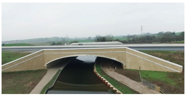
Heysham to M6 Link - Milestone Canal Bridge(654BI) (BEBO Arch T94S - Span 28.651m - Rise 3.213m)
